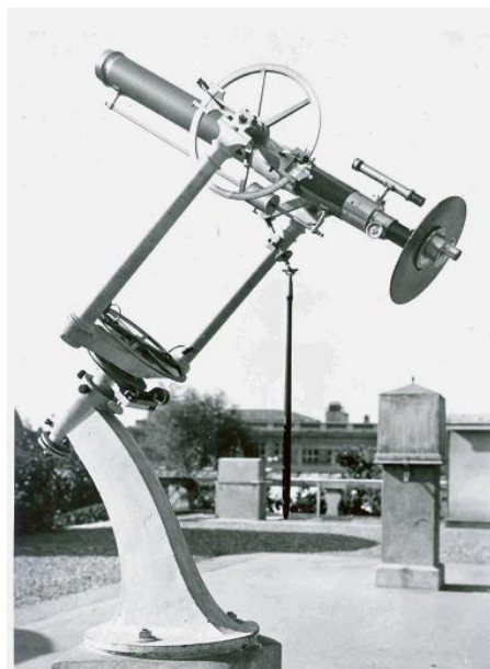
Figure 7: The Standard 83mm Fraunhofer refractor set up on the main terrace of the Observatory of Zürich (Source: Rudolf Wolf Gesellschaft, Bern; http://www.wolfinstitute.ch ).
